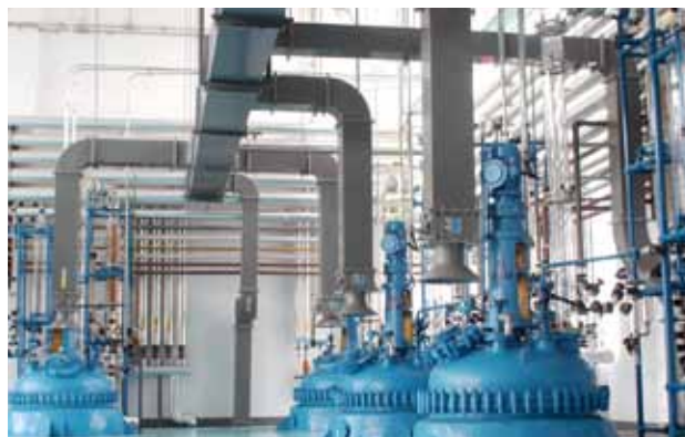
Pilot Plant Area I
